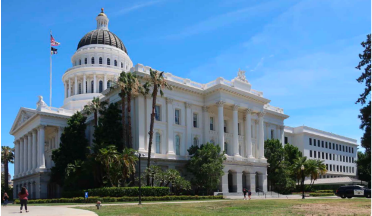
Photo by Preservation Architect Mark Hulbert
